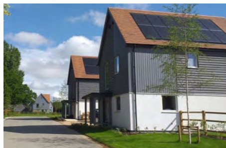
Wimbish, Passivhaus certified. (Source: Hastoe Housing Association)
